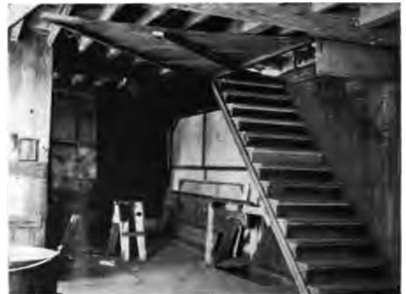
Fig. 5. Hinged Stairway Enclosure, raised.
